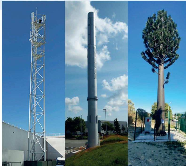
To blend them into any environment and safeguard the quality of its assets, Next Tower offers four types of tower: traditional lattice towers, as in Saint-Jean-de-Luz; monotube structures to conceal antennas, as in Orléans Saint-Mesmin and Brest Iroise; and even towers that resemble trees, as in Port-de-Bouc.
